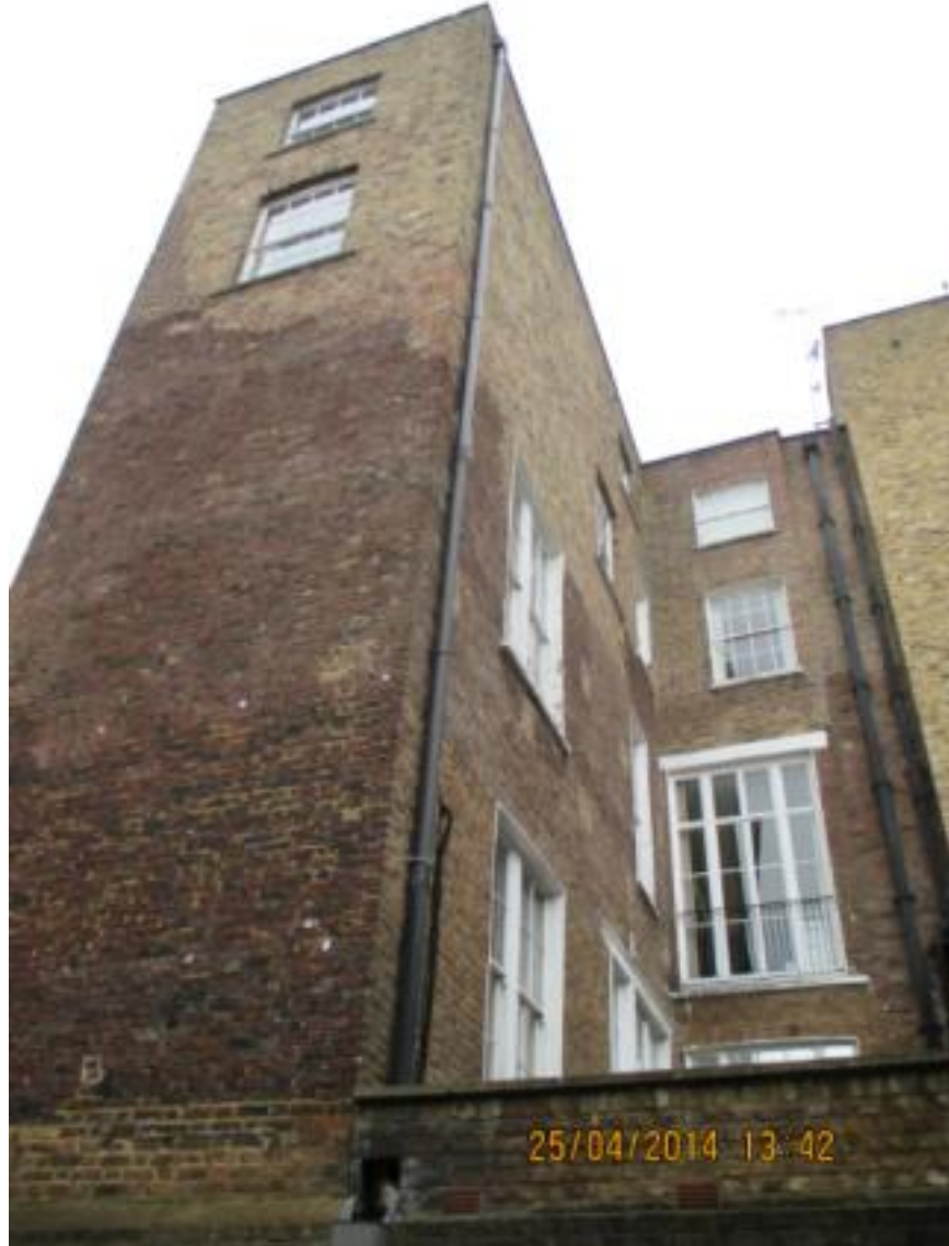
Photograph 3. Rear elevation of 93 Gloucester Place
