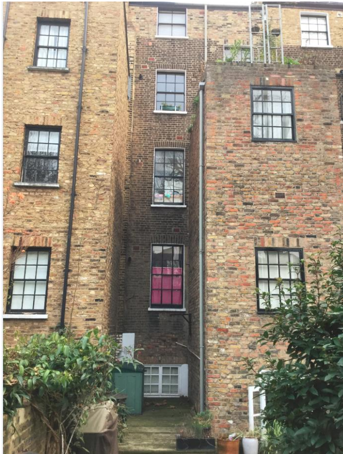
Rear Elevation & rear entrance Doors to lower Ground floor.
