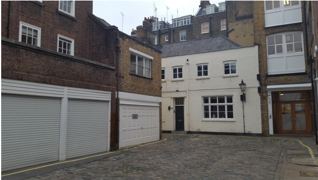
West elevation, facing Wigmore Place
