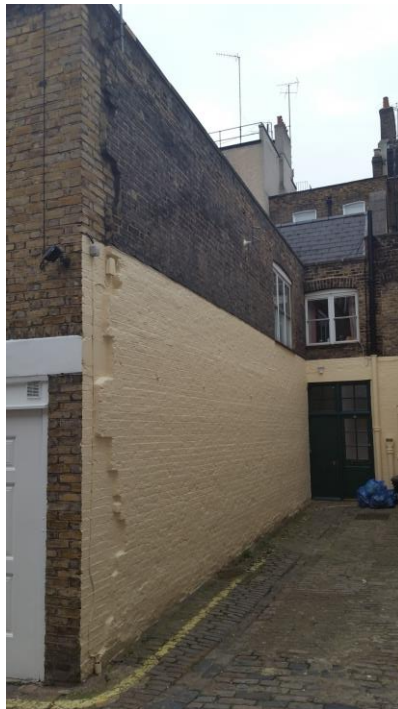
North elevation, facing Wigmore Place
